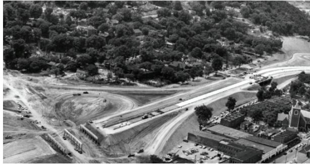
Photo: Golden Gateway under construction
