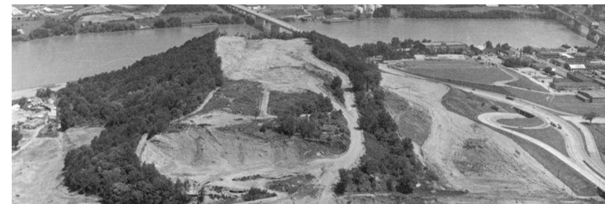
Cameron Hill during urban renewal, cut and fill for the highway
