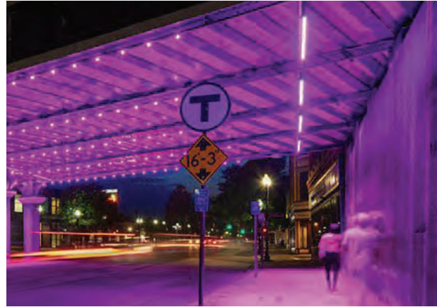
Underpass improvements with artistic lighting installation
